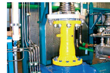
Gas turbine installation
